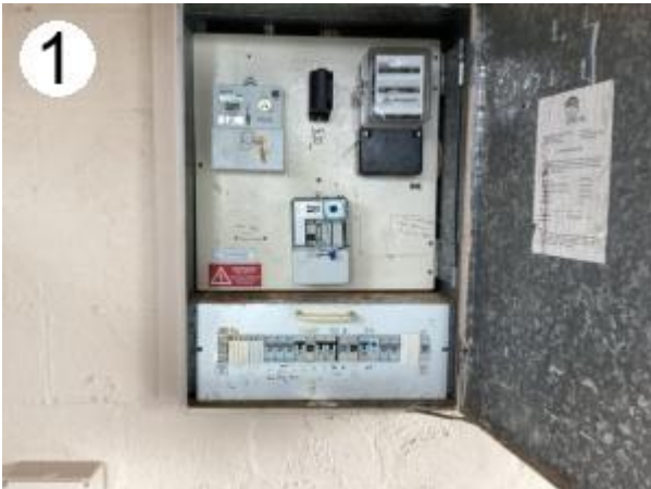
#1. A safety switch has been installed.
